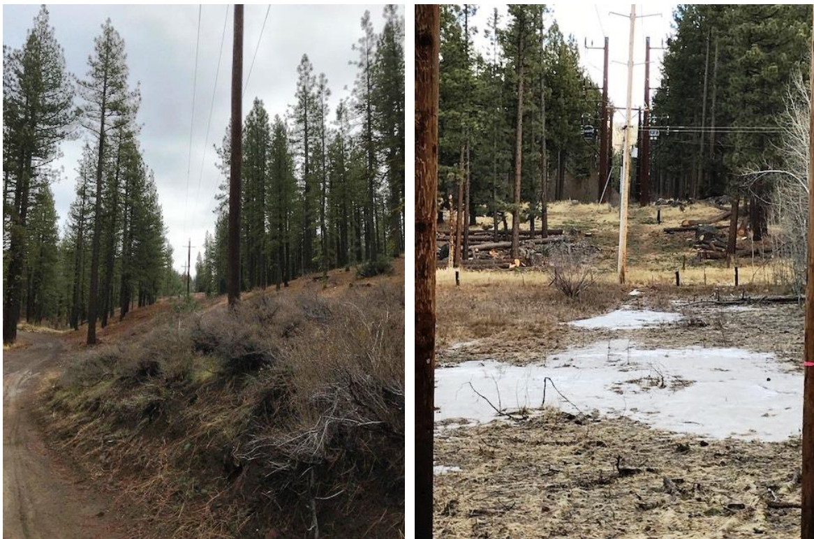
Figure 4-1. Example of Cleared Right-of-Way Floor on the Liberty Utilities Distribution System.
